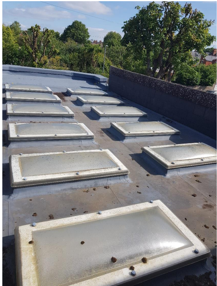
Figure 6 General view of the nave roof facing north towards the chancel. This roof is covered with a proprietary single-ply membrane and appears to have been renewed relatively recently.
