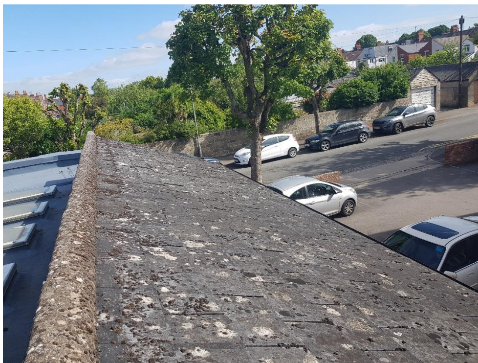
Figure 8 General view of the east aisle roof covered with artificial fibre (possibly asbestos-containing) reinforced cement slate. If not already carried out, an asbestos survey should be completed before carrying out works likely to disturb this roof.
