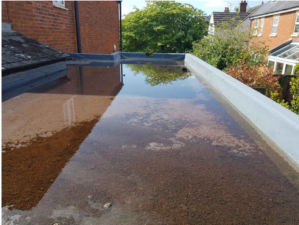
Figure 9 General view across the flat roof. The rainwater outlet was blocked causing ponding of water on the roof, which was cleared during the inspection
