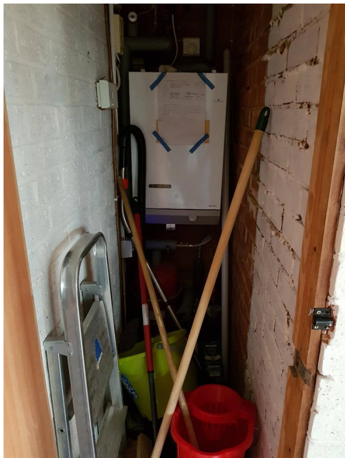
Figure 16 View into the janitor's cupboard within which the central heating boiler and heating controls are located. Access to the heating controls is difficult when the cupboard is full.
