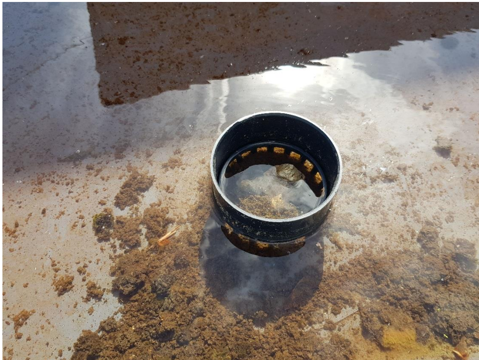
Figure 10 Blocked outlet to the flat roof above the entrance hall/toilet, this outlet should be checked/cleared regularly.
