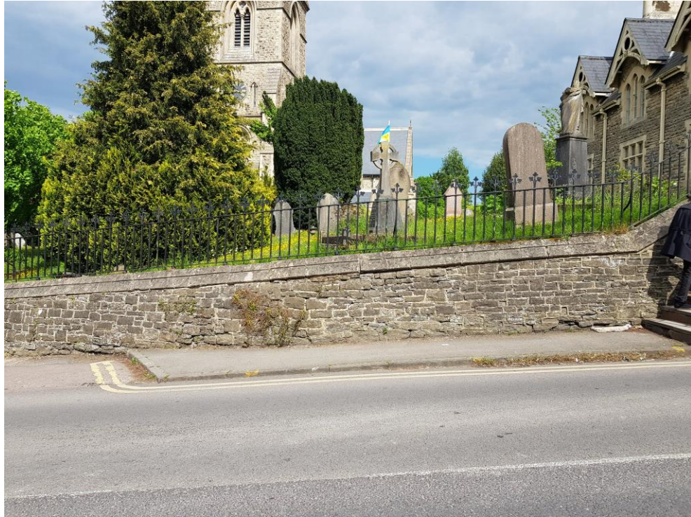
Figure 19 General view of the church and the west boundary wall from the public highway; this boundary wall has a number of missing/loose stones and the pointing/bedding to the rubblework is generally in poor condition. Repairs to the wall would be prudent within the next quinquennium
