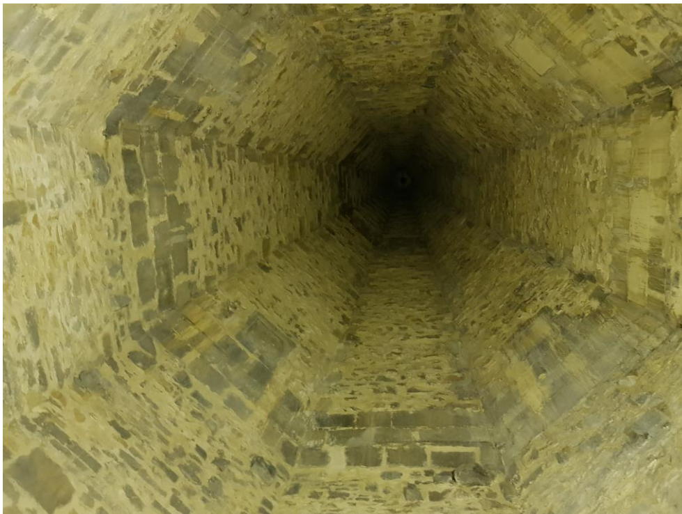
Figure 10 General view of the underside/interior of the spire as viewed from the deck at the base; the spire interior was dry at the time of inspection, however it was reported by the churchwarden that water ingress through the spire masonry remains an issue
