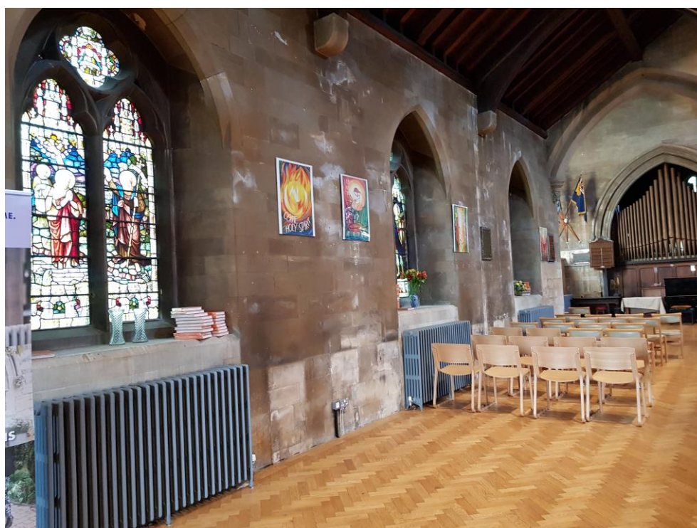
Figure 16 General view of the north wall of the north aisle showing salts related staining and ghost-marks where previously fitted pews have been removed
