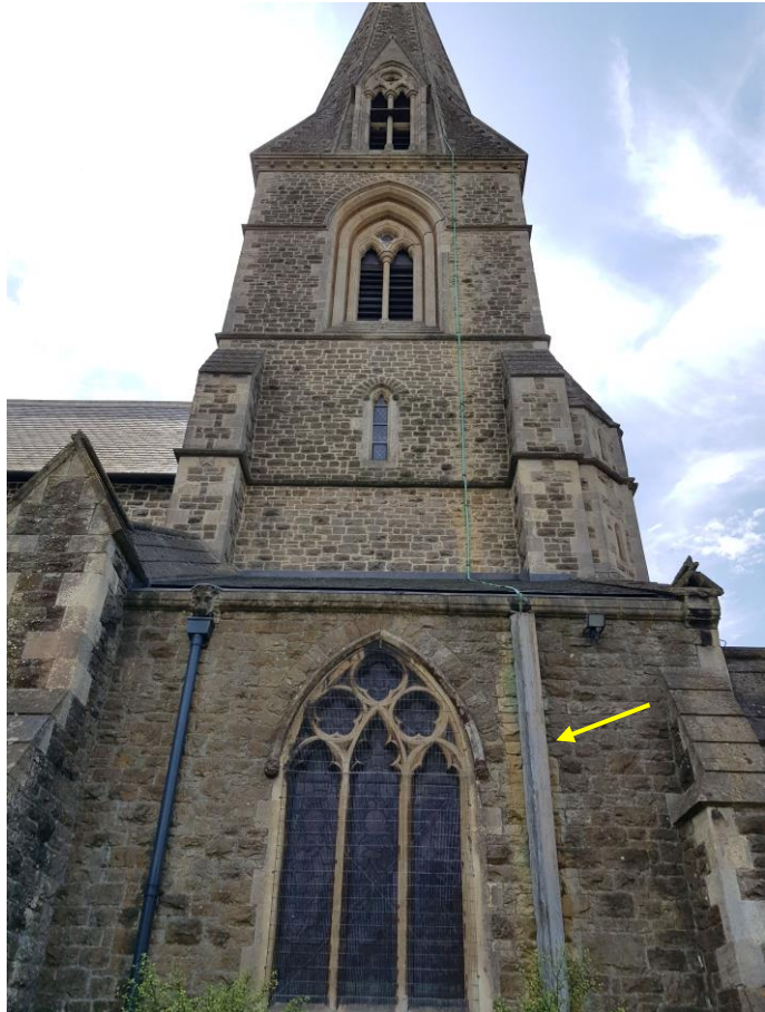
Figure 5 View of the tower north side showing timber casing to the lightning conductor tape; presumably required for insurance purposes. The casing is unsightly and, at the very least, would benefit from redecoration
