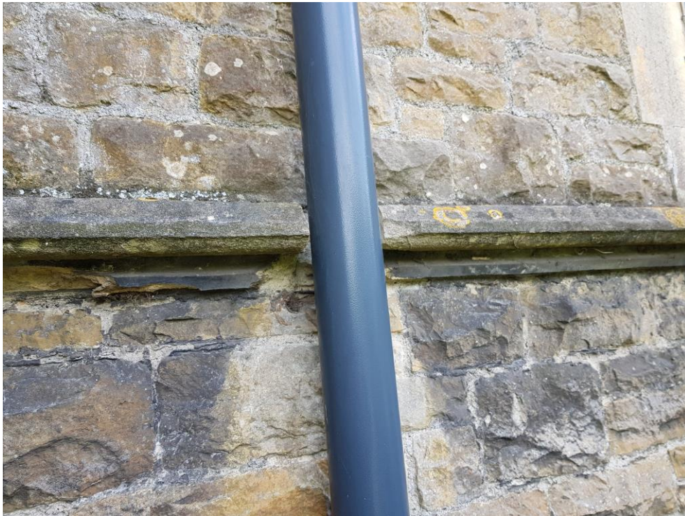
Figure 7 Example of where a string course has been cut through to allow fitting of rainwater goods, presumably carved out as part of the recent overhaul of the chancel roof carpentry and rainwater disposal system
