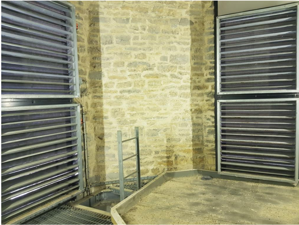
Figure 11 General view of the spire interior showing the main-deck and internal, electronically-operated baffles fitted to each of the tower belfry openings
