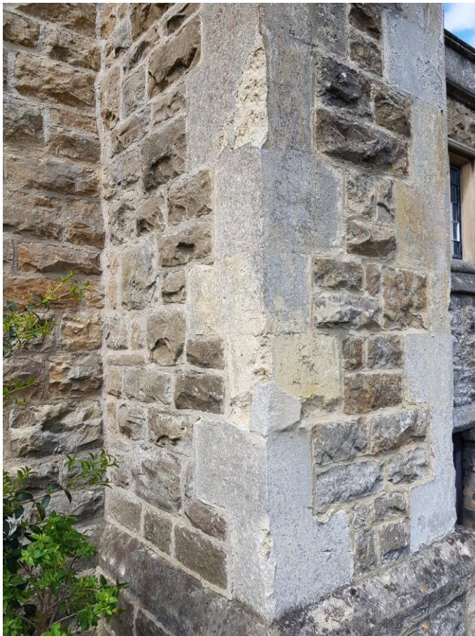
Figure 6 Detailed view of the buttress to the north-east corner of the chancel, which shows ‘soft bed’ erosion and surface decay to the stonework, typical examples of decay to ashlarwork found throughout the church externally
