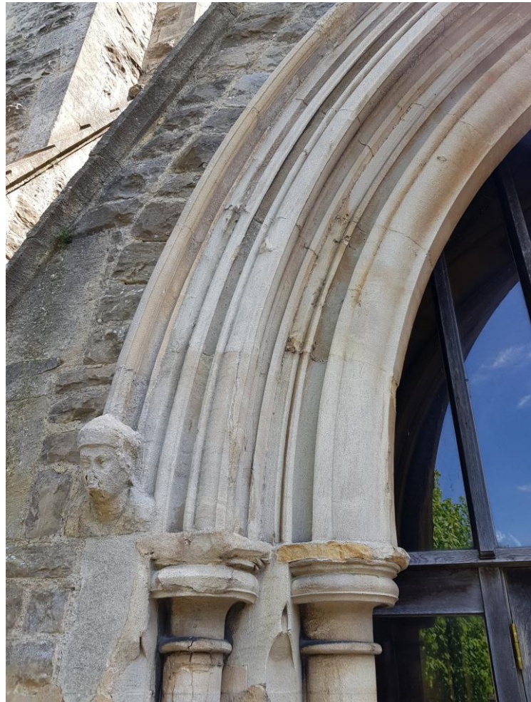
Figure 9 View of the left-hand springing point to the external arch of the west door showing extensive decay to dressed and carved limestone ashlarwork, together with previous mortar repairs now succumbing to decay; these repairs were originally intended as sacrificial to protect the stonework to which they were applied). Renewal of mortar repairs and other conservative repairs to external stonework would be of considerable benefit to conserve the church fabric within the next quinquennium
