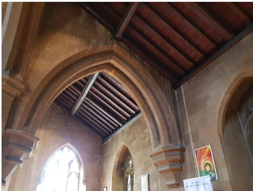
Figure 15 General view at the west end of the north aisle interior showing staining to stonework from previous ingress through the roof, presumably prior to renewal of the roof coverings
